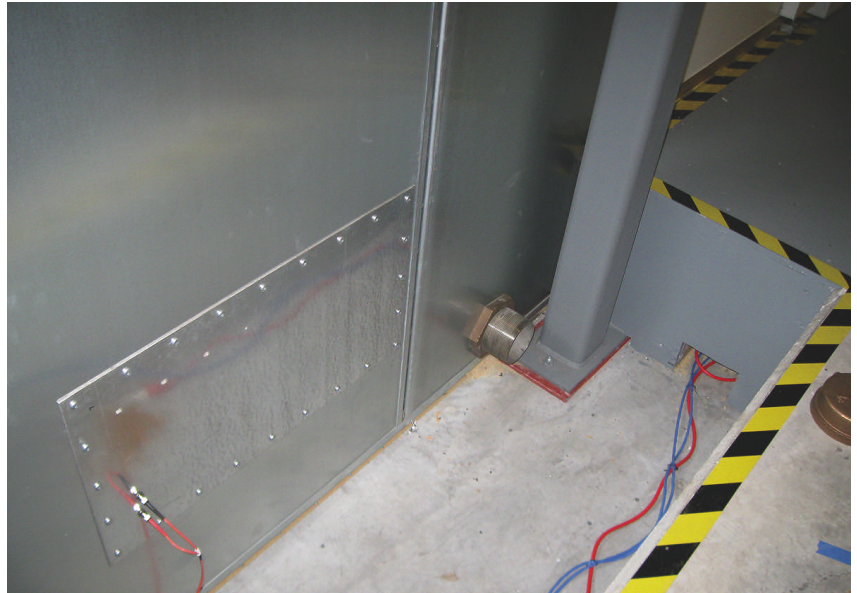
Figure 4 A penetration panel sits below the building floor, providing access to cables that run under the chamber's raised floor. A pipe opening alongside the panel provides access for additional cables and hoses (courtesy Northwest EMC).
